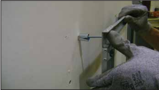
Figure 4.6 Installing Anchors in Hollow Wall
