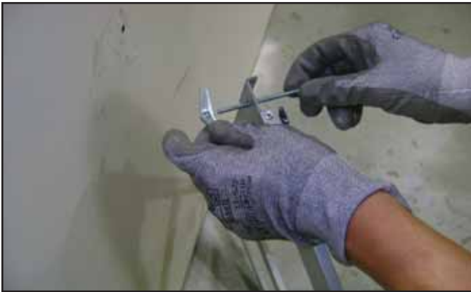
Figure 4.5 Toggle Bolt Installation through Mounting Bracket
